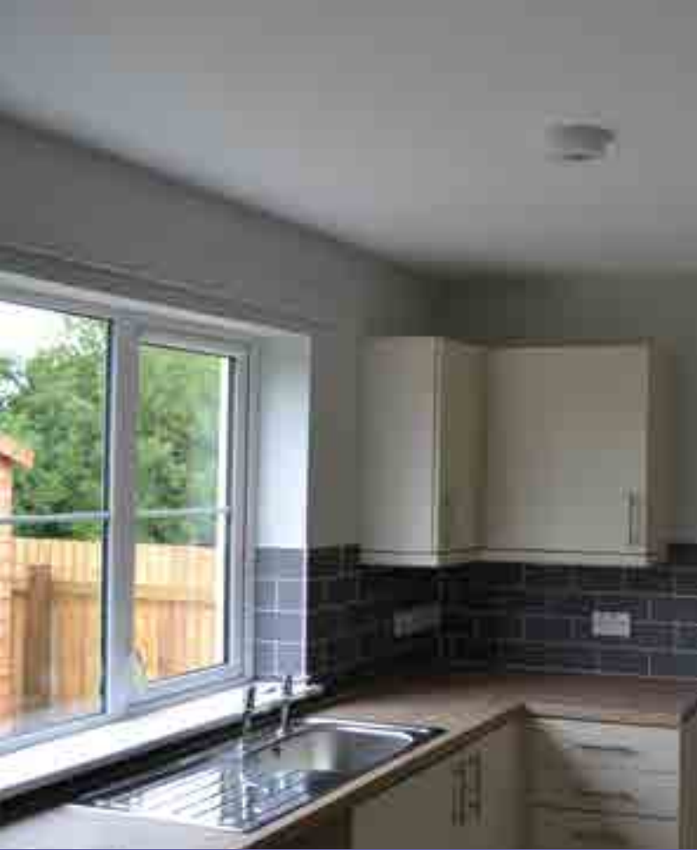
Quality workmanship at Llantilio Crossenny
