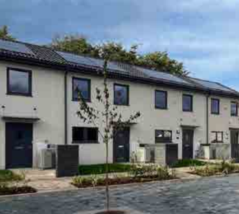
Solar panels at Juneberry Drive, Bulwark
